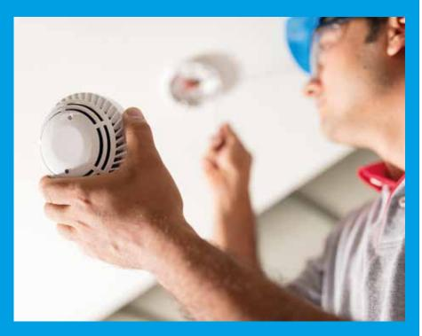
We will install a smoke alarm in each circulation space within your home and within the room you use the most. This usually means hallways and living rooms. We also fit heat detectors in the kitchen and all alarms are interlinked.
